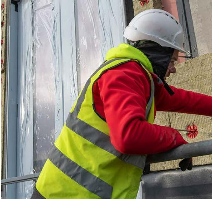
The team utilised ROCKWOOL RainScreen Duo Slab because of its [Euroclass] A1 non-combustibility and its proven thermal and acoustic qualities in addition to being a well-known and trusted brand for this type of project.
